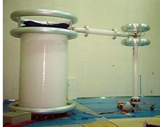
Test system 350 kV, 2 A with damping resistor
